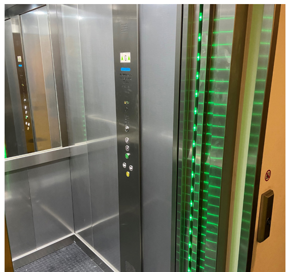
New lift interior and door detector edges
