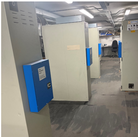
The lift control panels.
