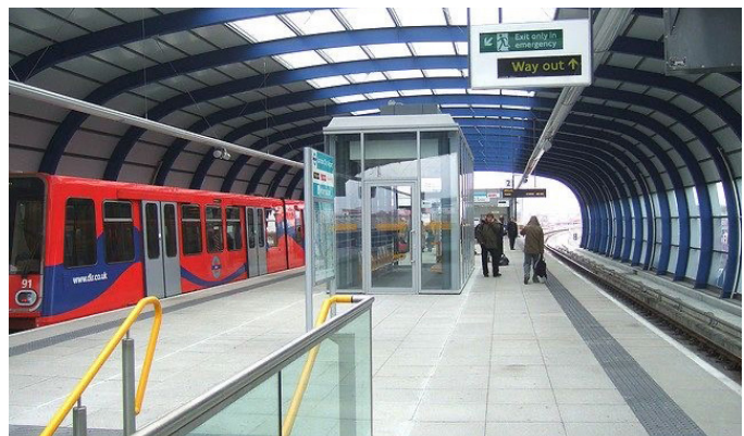
A modernised lift at one of the twenty DLR stations
