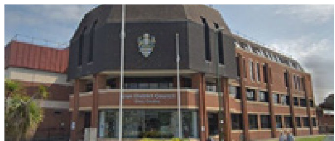
Arun District Council's Civic Centre
